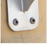
Stainless steel screws and/or screws covered with plastic caps,
